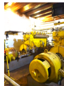
Subterranean Electricity Generator for Fort
