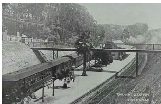
Warrawee Station at the time of the accident
