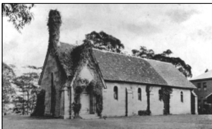
The photo is of the St John's after the 1899 extension. The smaller original church was understood to have been incorporated into the 1899 extension (see the lighter roof colour). This section remains today.
